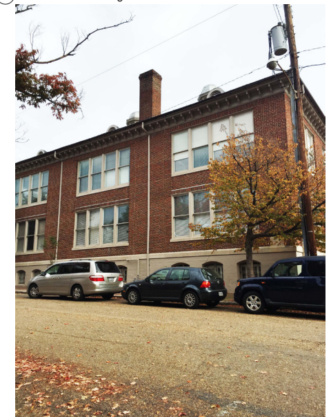
④ View to the building from intersection
