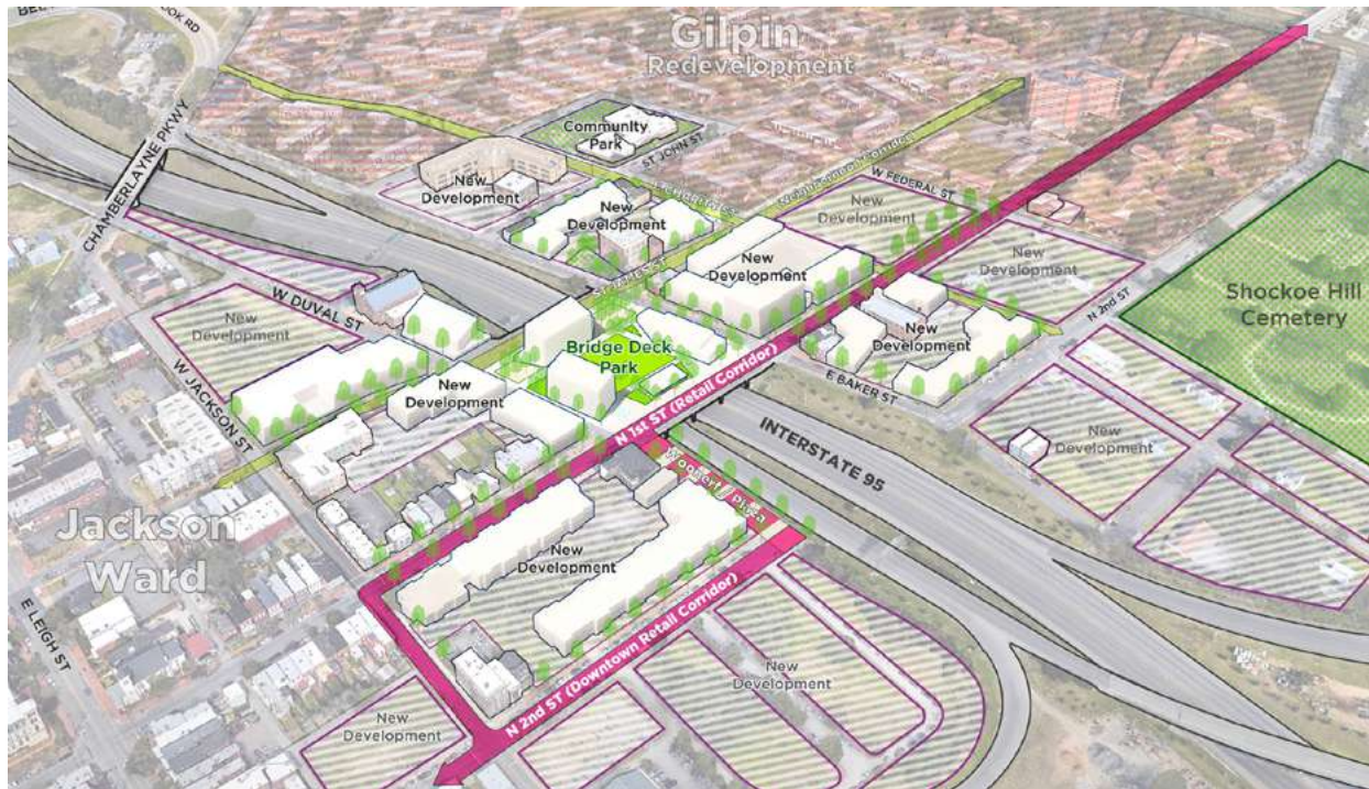
Jackson Ward Bridge Deck. By capping the highway between Jackson Ward and North Jackson Ward with streets, parks, and buildings, Jackson Ward will once again be one neighborhood. Credit Richmond 300: A Guide for Growth.
