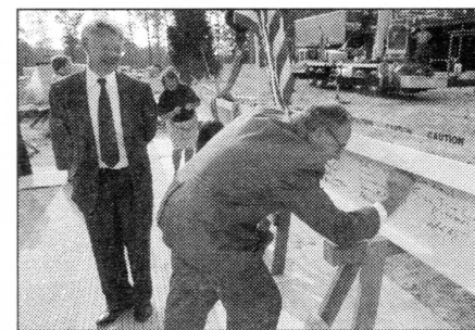
Once signed by all the attendees, the final steel beam was raised to the roof of the structure.
