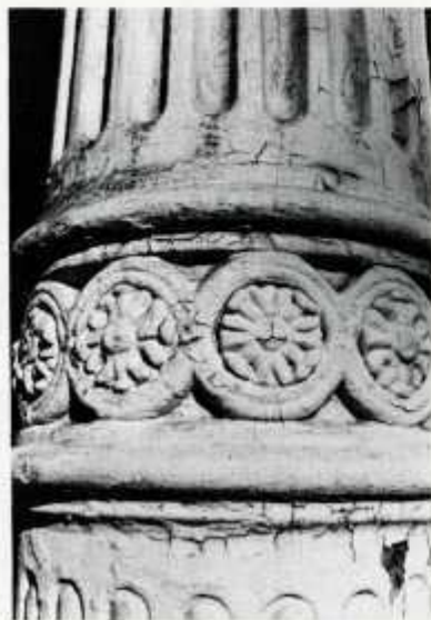
Details of columns at front of Founders Hall. Photograph from the November 1972, "VCU Mag- azine," by Robert Hart.
