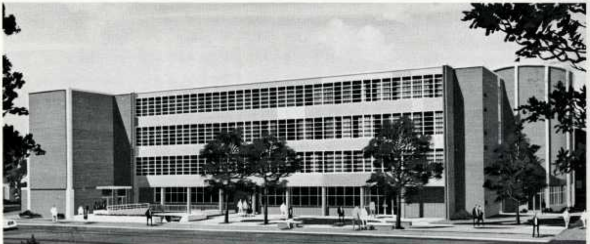
The Hibbs Building after both wings were completed.
