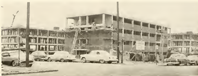
New Dormitory Progresses
