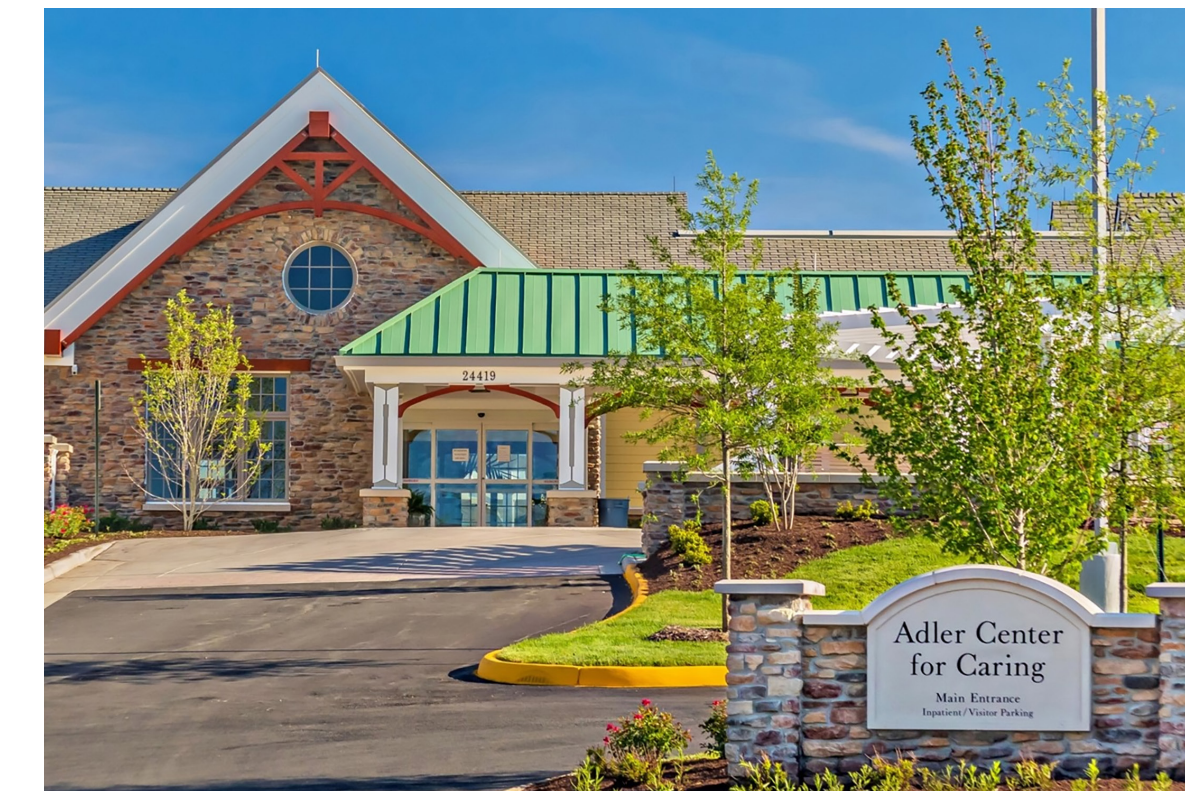
Entrance to Adler Center for Caring
