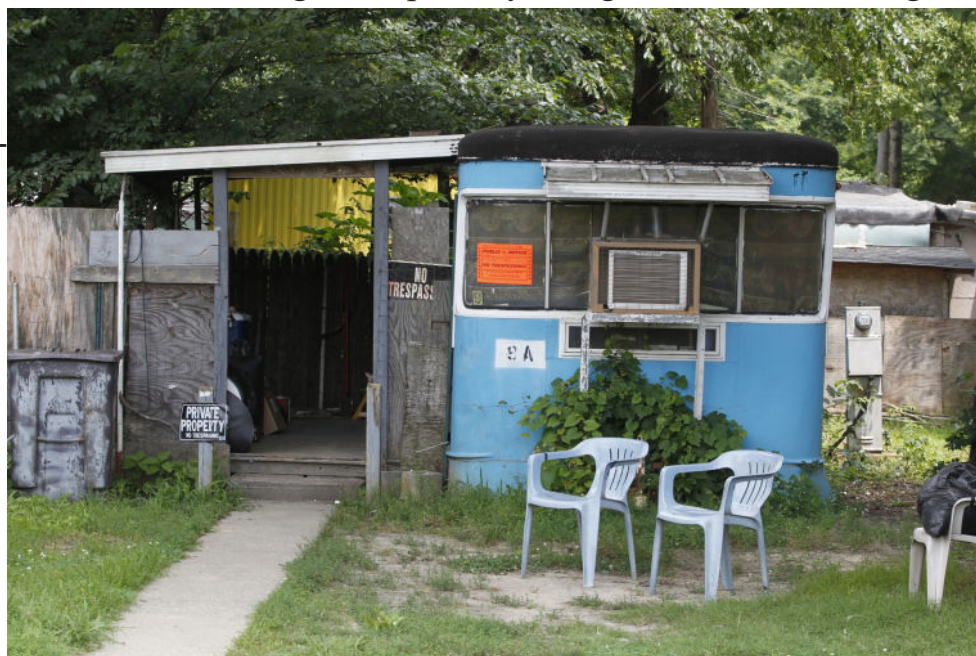
Building code violation posted on a home in Rudd’s Trailer Park
