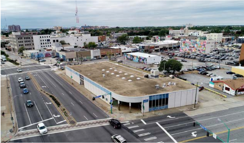
Figure 45. Former Greyhound Bus Station at the corner of Brambleton Avenue and Monticello Avenue in Downtown Norfolk
