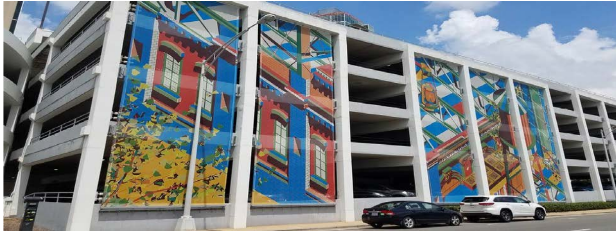
Figure 46. Parking Garage with artwork display, Durham, NC
