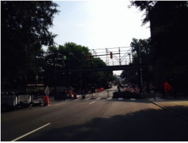
Day two of pedestrian bridge construction shows is underway.
