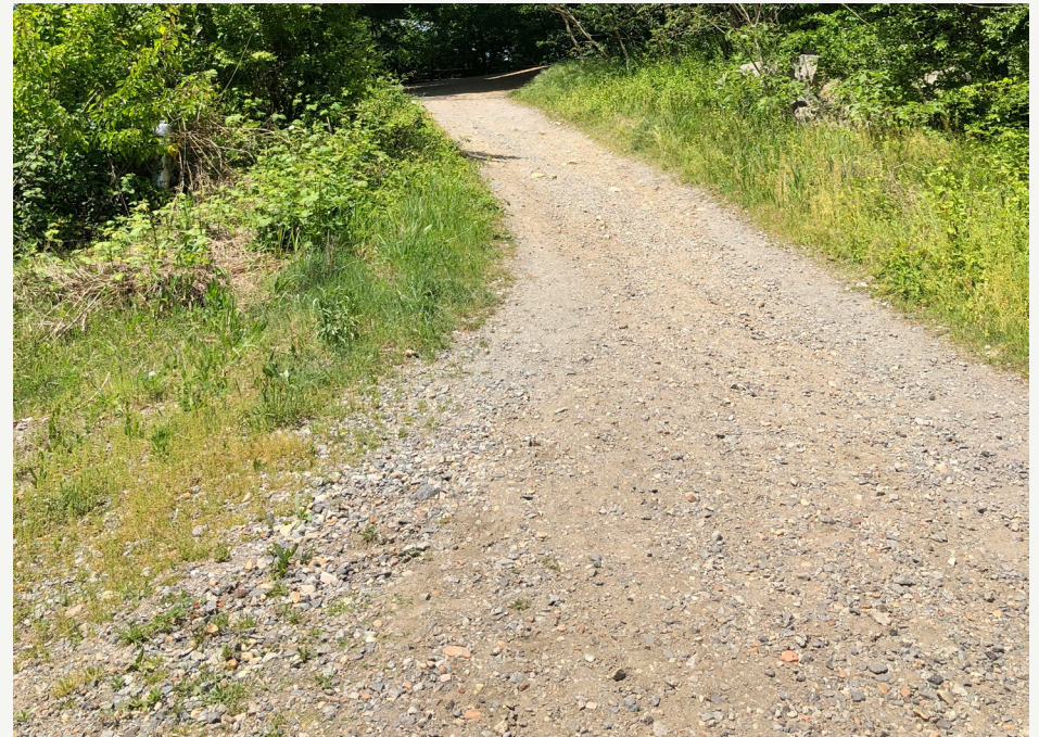
Figure 49 | Unpaved pathway connecting Oregon Hill, North Bank Trail, and Tredegar Street
