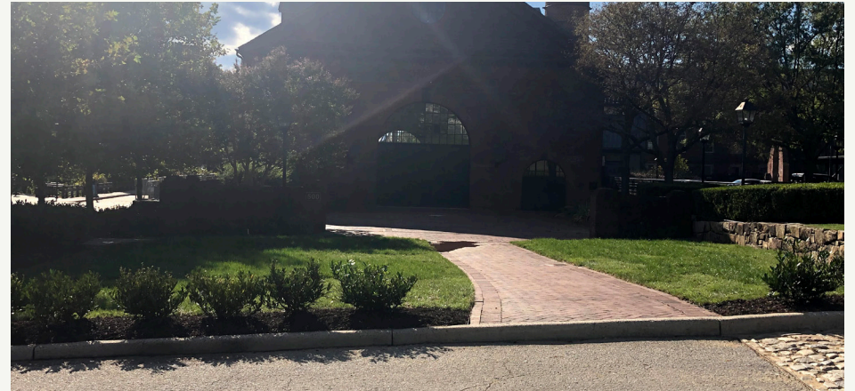
Figure 17 | Westbound, no curb ramp on sidewalk heading towards ACWM
