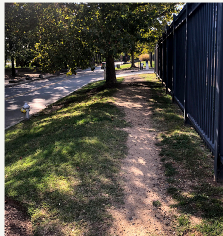
Figure 16 | Westbound, unpaved sidewalk conditions next to ACWM Parking Lot
