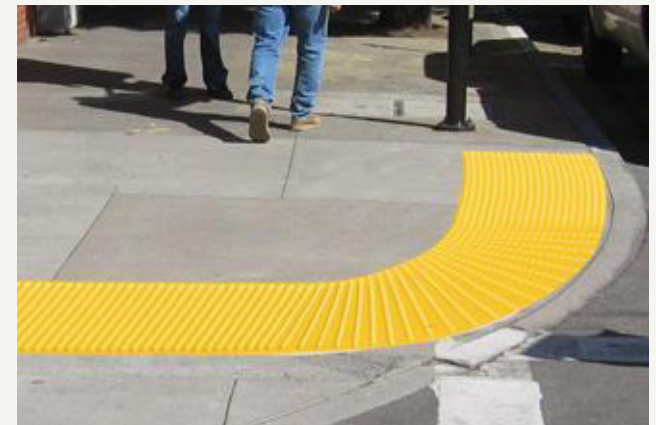
Figure 47 | Detectable warning surface
