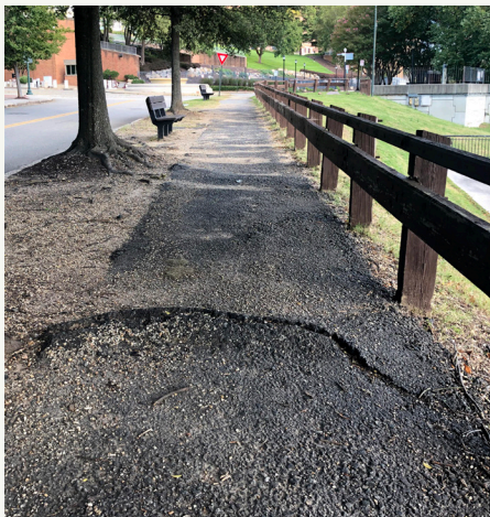
Figure 15 | Eastbound, uneven sidewalk conditions across from CoStar Building
