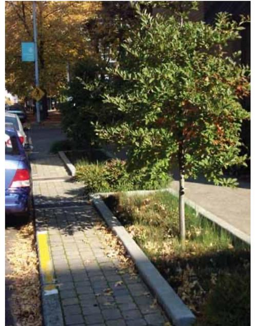
**Figure 26. Continuous or linear planters or swale within sidewalk**
