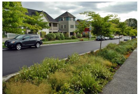
**Figure 27. Continuous swale extended from curb with crossing**
