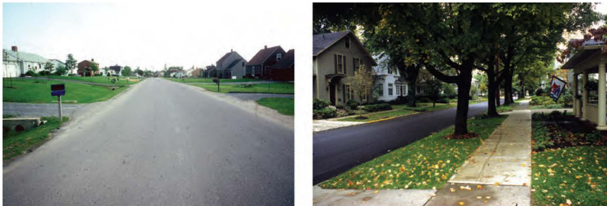
Figure 2-4: Modern subdivision standards have created a building form completely out of scale with historic development patterns of older settlements, with distances between opposing house fronts literally double that usually found in traditional neighborhoods. Shown on the left is a typical rural subdivision of conventional design with wide streets and deep front setbacks in Middlebury, Vermont. People living on opposite sides of the street often hardly know their neighbors. By contrast, traditional streetscapes with appropriately scaled road pavement and modest front yards or “dooryard gardens” grace many older communities such as Granville, Ohio (right), where sidewalks and shade trees add to livability. (Source: Randall Arendt)
