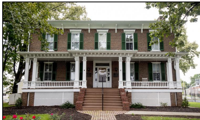
Image J. Jennings House, courtesy of Lantz Construction.
