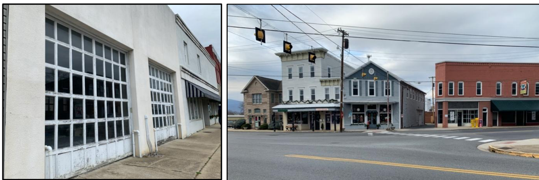
Images E (left) Downtown Building in Need of Repair. Image F (right) Downtown Storefronts and Vacancies.
