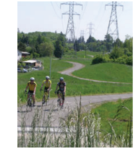
Figure 39: Example of a bike path below power lines
