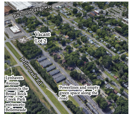
Figure 38: Overview shot of the Bellemeade-Richmond Highway corridor showing the open space under powerlines
