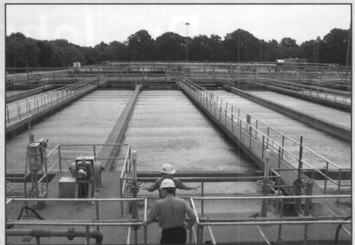
Dr. Richard Roadcap Views Hopewell Treatment Facility. Watch for your BMP manual!
