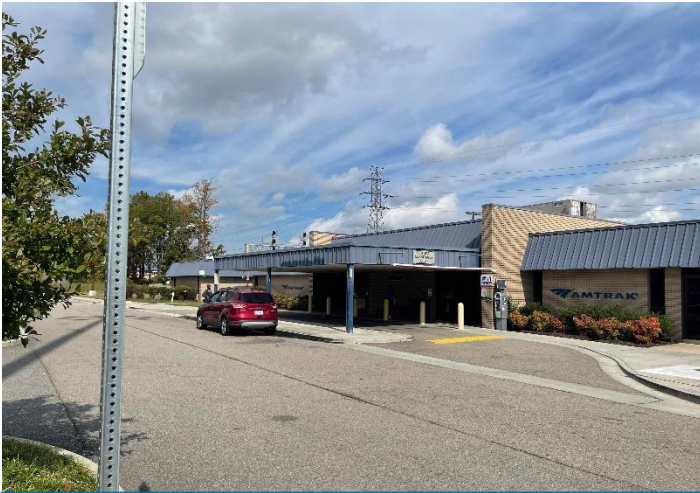
Amtrak Staples Mill Station Entrance
