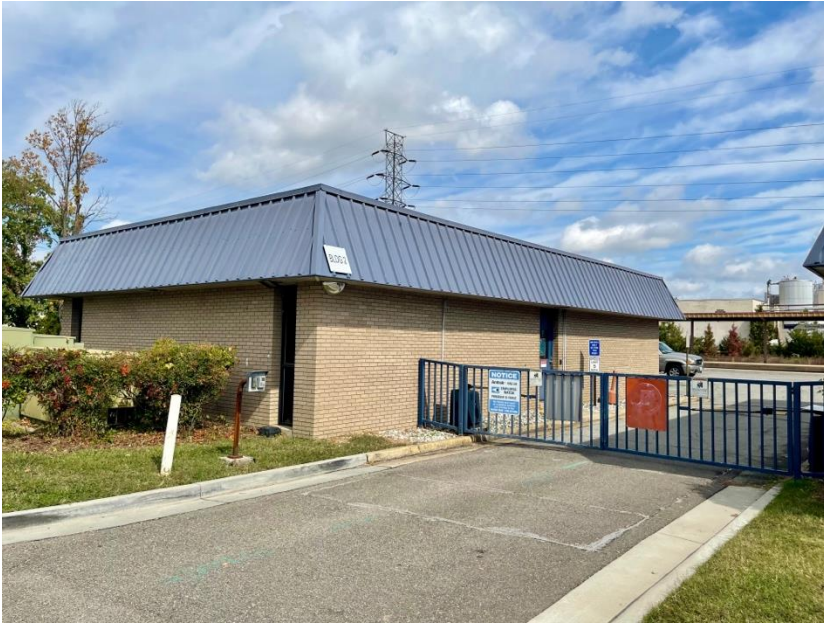
CURRENT STAFF OVERNIGHT ACCOMMODATIONS (INADEQUATE)
