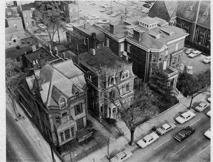
Site where Rhoads Hall now stands. The old Pace church stands beside it.
