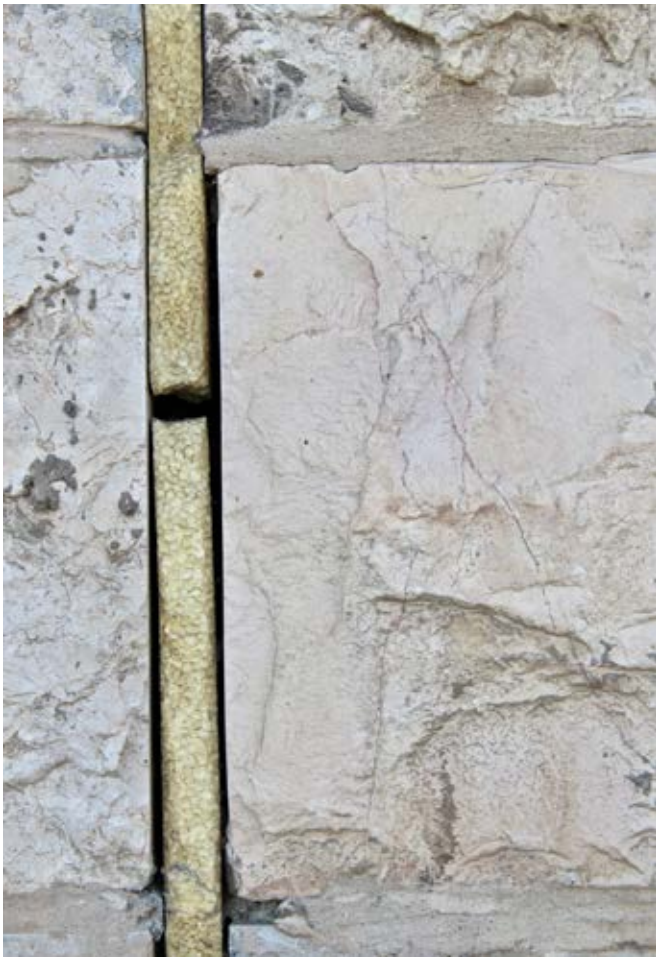
Figure 7. Styrofoam Between Cinderblocks
