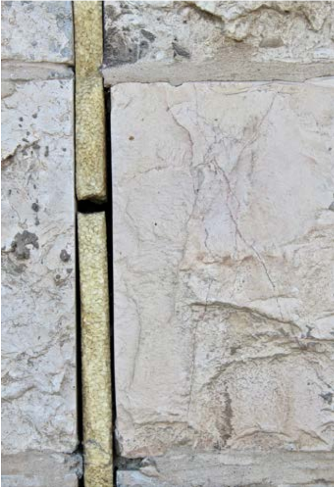
Figure 7. Styrofoam Between Cinderblocks
