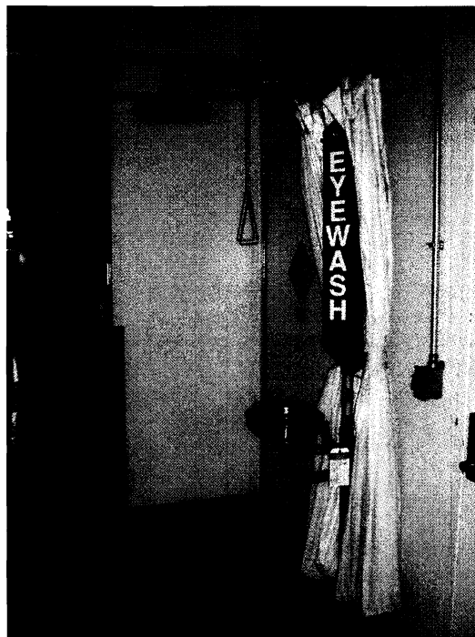
Figure 2: Combination eyewash and shower station
