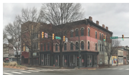
122-124 E BROAD STREET, BUILDING EXTERIOR
