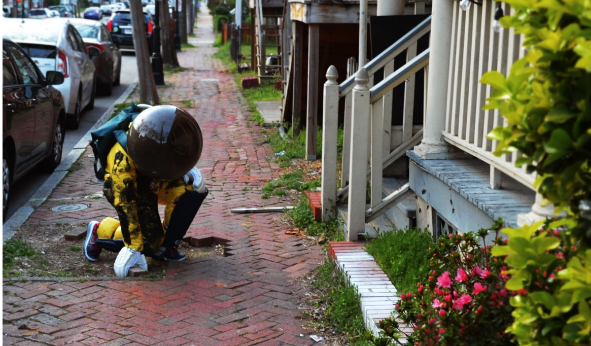
Picking up bricks in OYA-9394. Richmond, Virginia.
