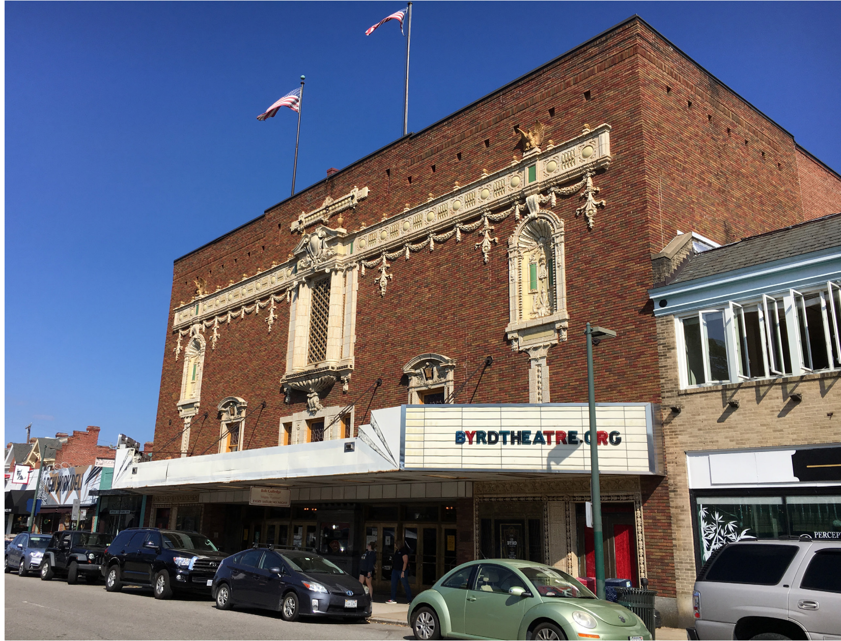
Fig. 72 Front Facade & Marquee
