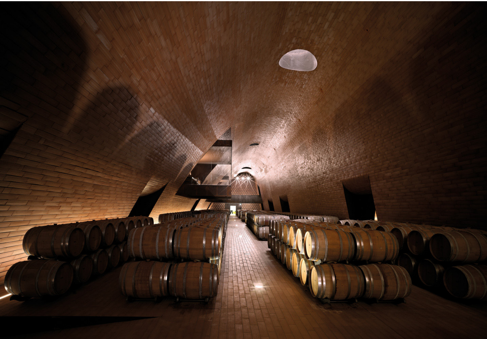
24.1 These double-height cellars are arranged in three rows and are lined with terracotta on every side.
