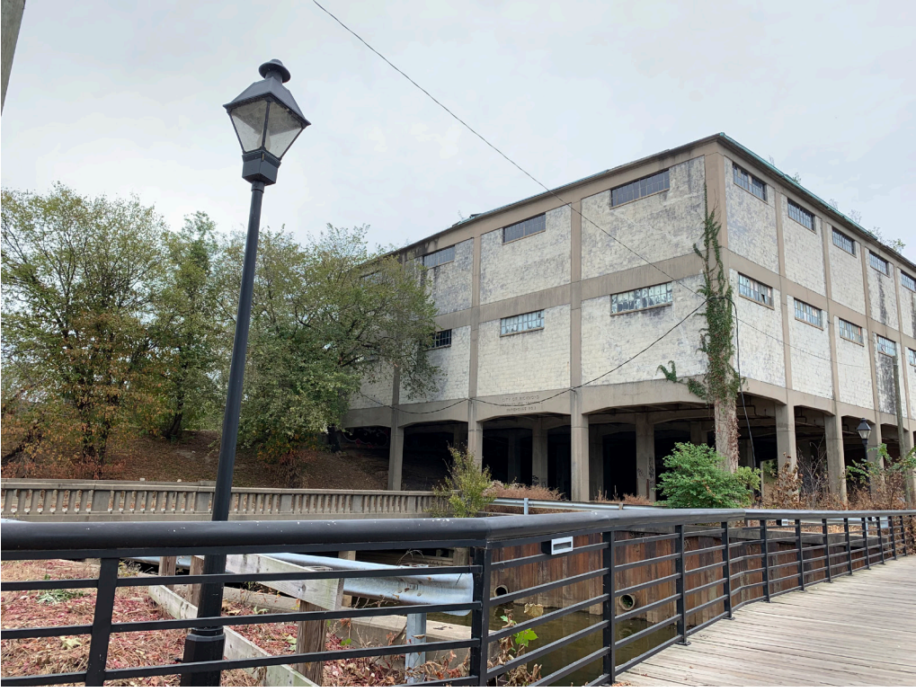
View B - From Bridge
