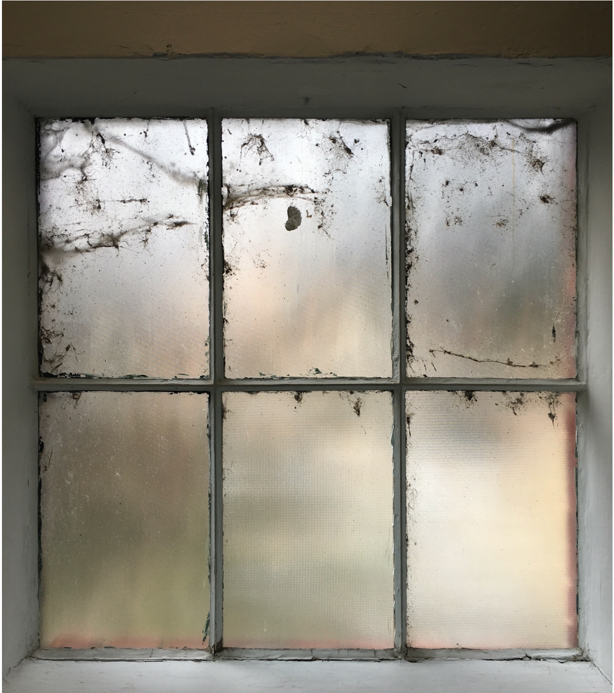
Figure 61. Picture of a window where the Landscape work will be installed
