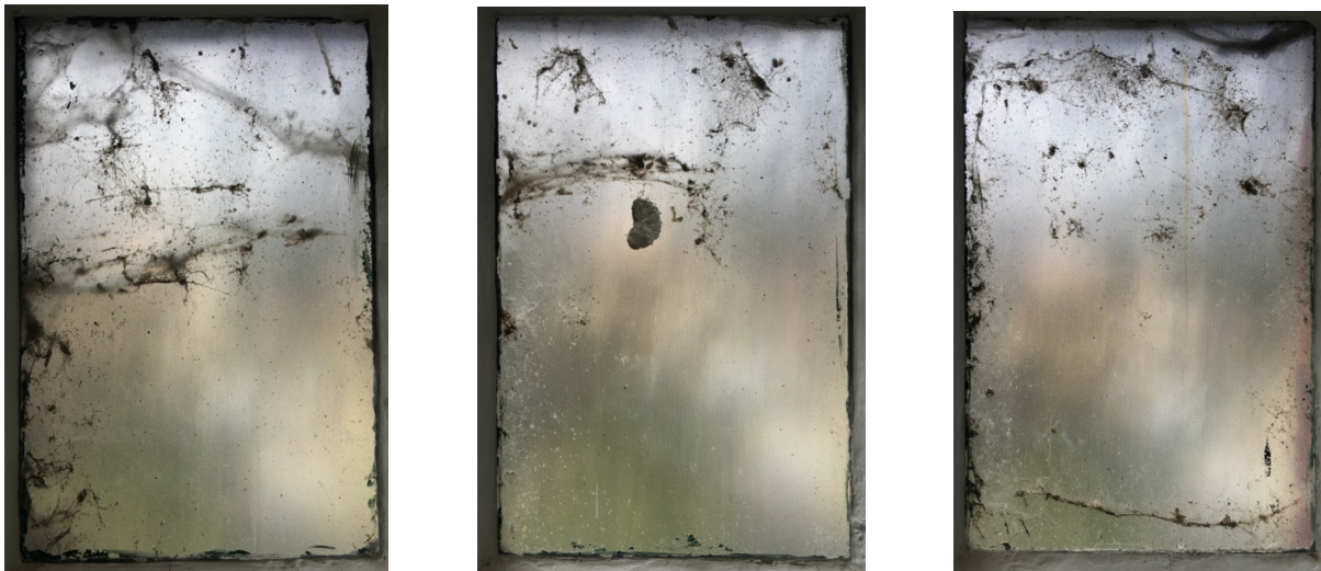
Figure 60. Picture of a window's detail where the Landscape work will be installed
