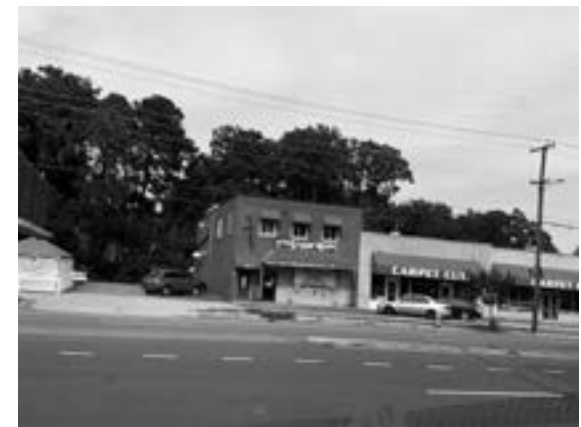
EXTERIOR - RIGHT ADJACENT BUILDINGS
