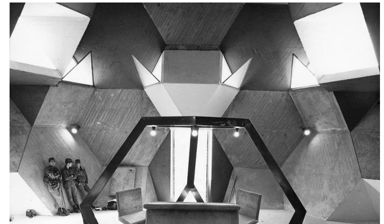
Fig. 7. Interior view of the Synagogue at the Officers School Training Base I, Israel.
