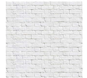
PAINTED BRICK Exterior Existing Walls
