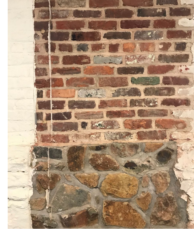
Stone foundation married into exposed brick
