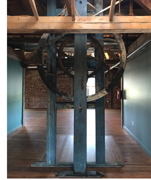
Original hoisting machinery with patched floor
