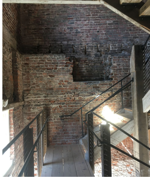
Original carriage house structure in stairwell
