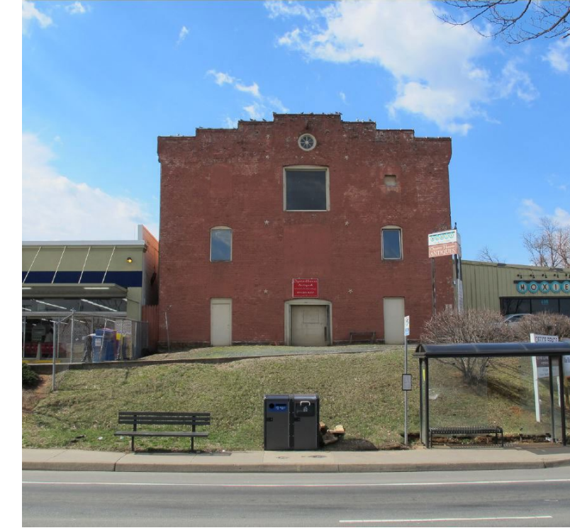
King Lumber Company facade prior to renovation (2015) photo courtesy of current building owner
