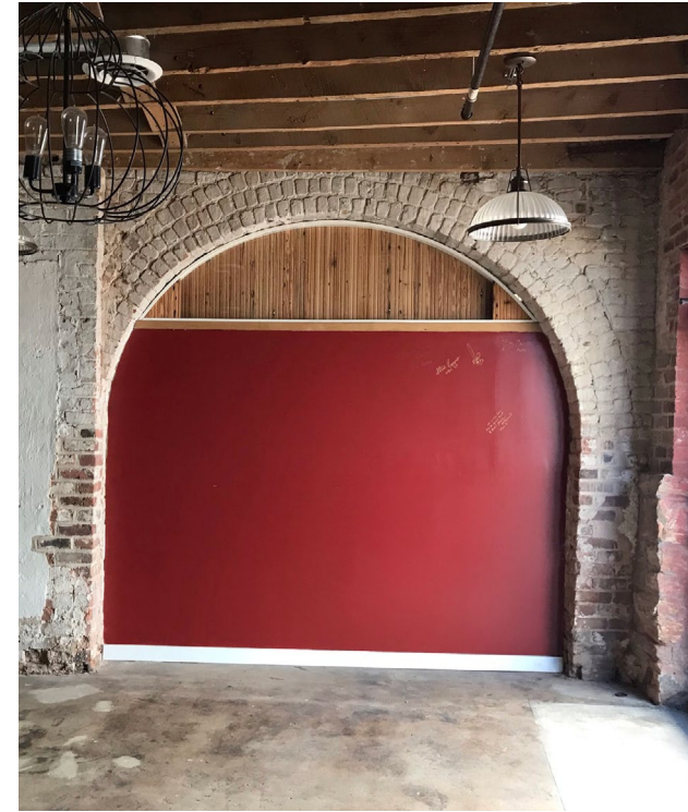
Filled carriage house door beneath existing stairs
