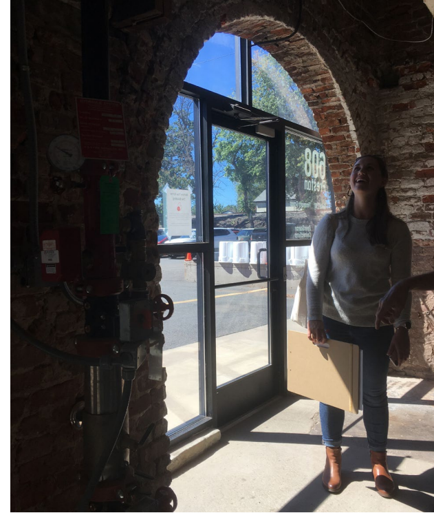
Inside exterior carriage house storefront solution, adjacent to existing stairwell
