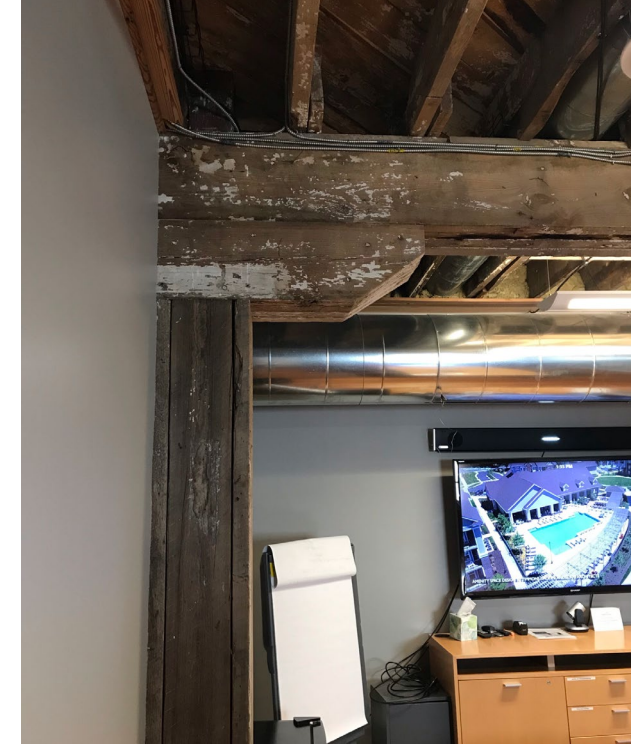
Exposed ceiling and heavy timber construction
