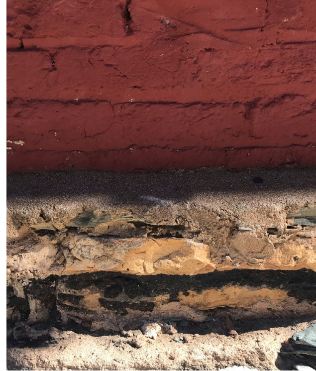
Close-up of rubble stone foundation
