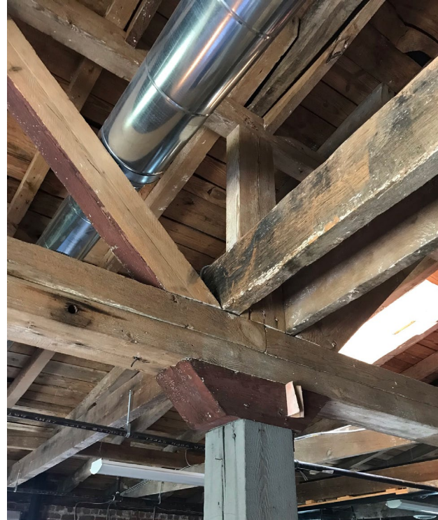
Exposed ceiling and heavy timber construction
