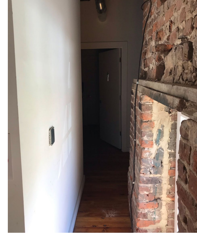
Existing elevator (left), south exterior wall (right)
