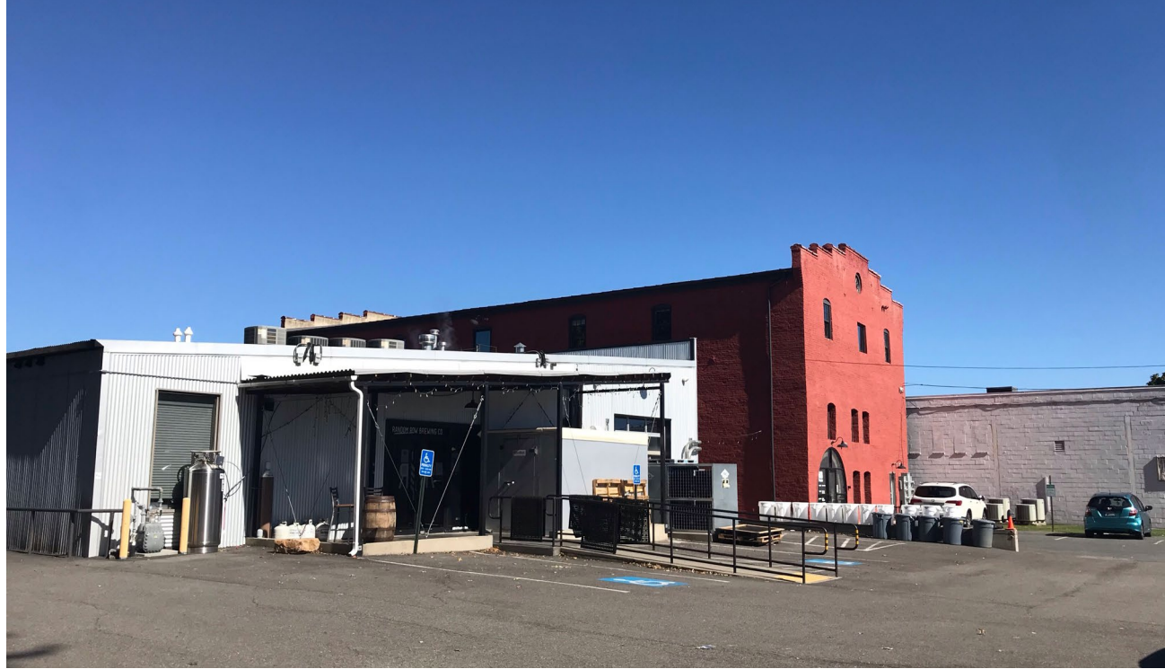
Facing east from the rear parking lot
