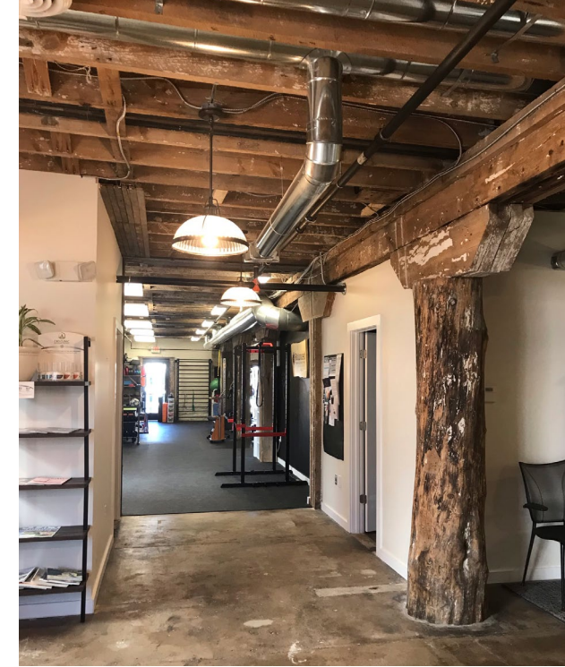
View from west breezeway entrance adjacent to filled carriage house door; tree column
