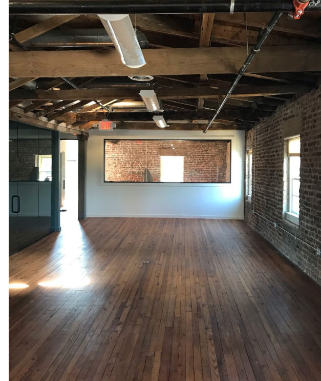
Facing south, view of existing interior window overlooking open stairwell
