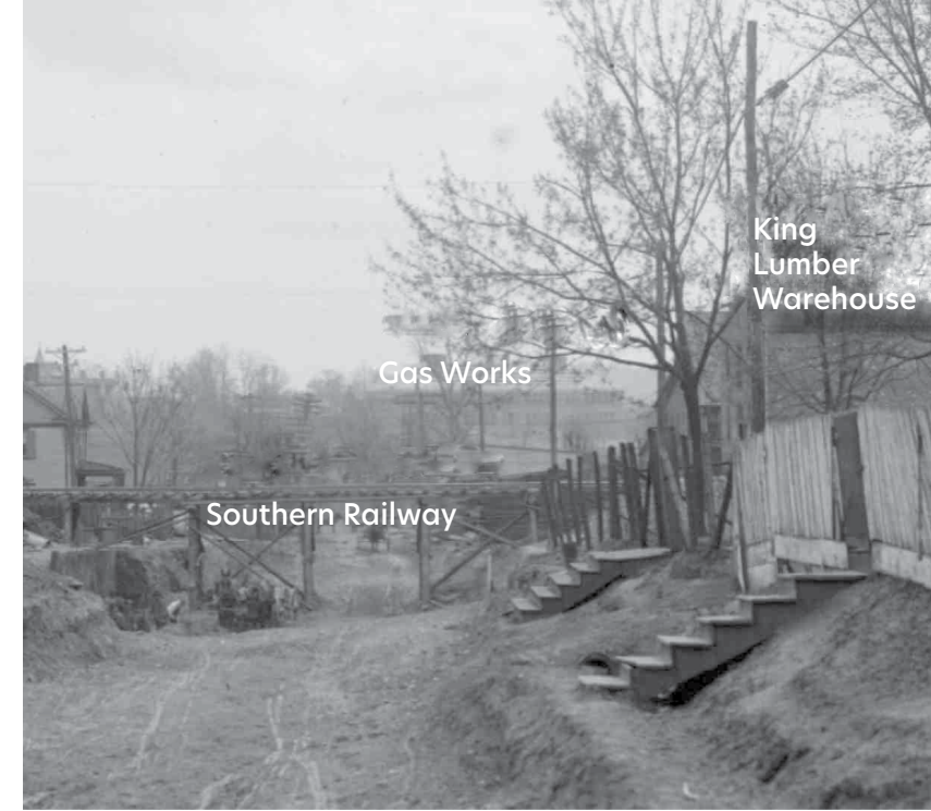
King Lumber surroundings after railroad overpass (date unknown) photo and annotations courtesy of Bridge Finder
