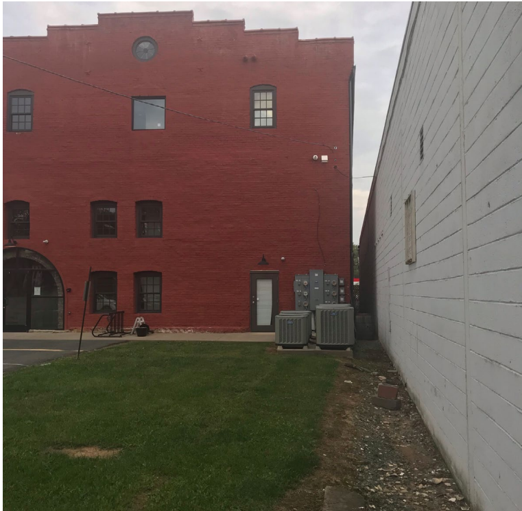
Reid Grocery Market obscures morning and midday sun from the east on the first floor of the King Lumber Building.
