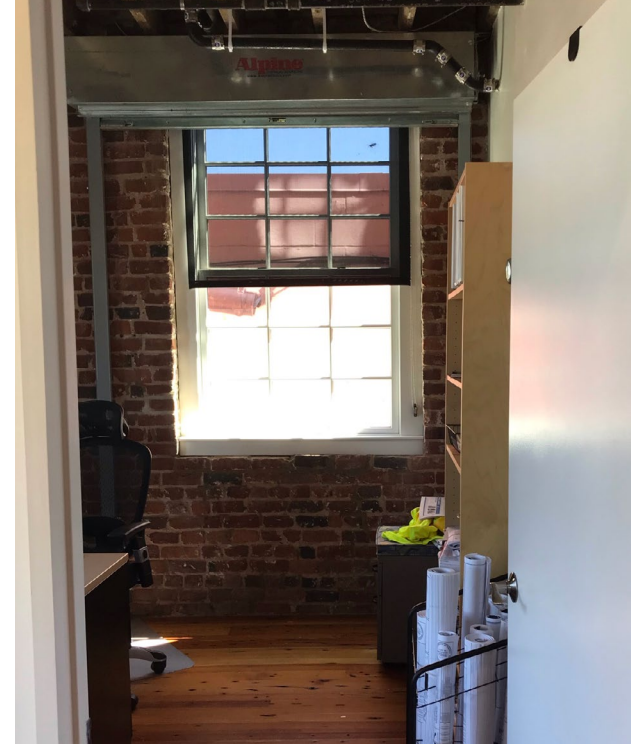
East-facing window partially obscured by market
