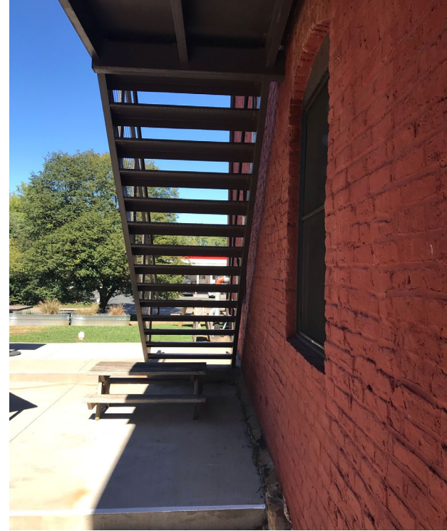
Stair access to three floors on east elevation
