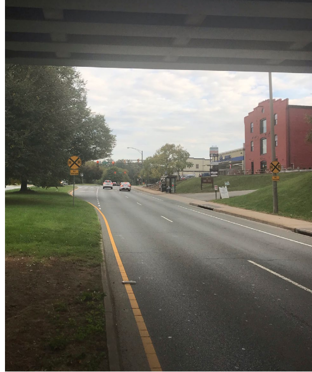
Facing east from Preston Avenue median under the Norfolk Southern / Amtrak train overpass
