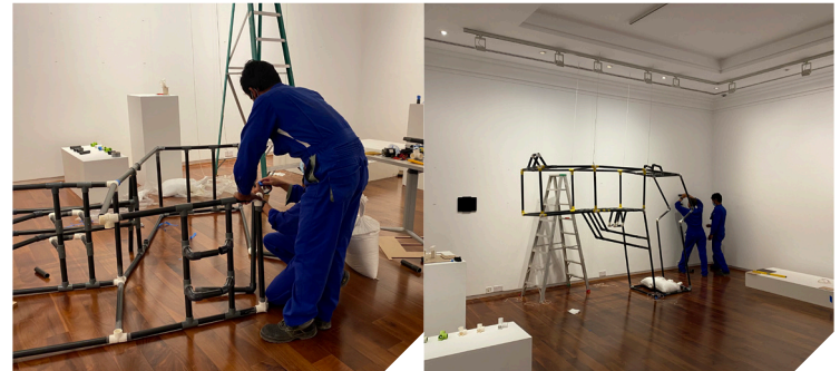
Figure 33. 3D printed joints, VCUarts Qatar, 2021
