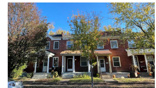
4 North view from the building
