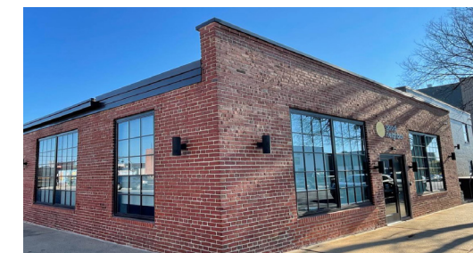
2 South view from the building
