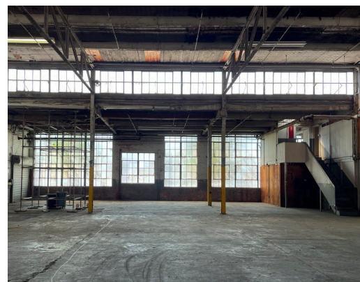
West Wall View
